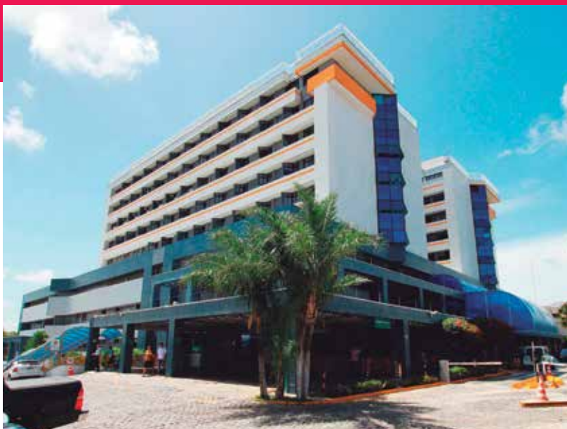
Hospital Regional Unimed Fortaleza
